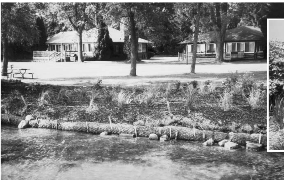
A newly installed shoreline restoration project using natural coconut fiber rolls to stabilize the banks and plantings along the riparian zone at the Sylvan Mounds II site. This project was installed in the summer of 2001. The native plants and shrubs require little maintenance, and will become fully mature within a couple years.
