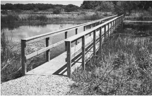
New boardwalk at the lake District Preserve.
