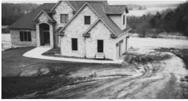
An active construction site on Lake Ripley.
